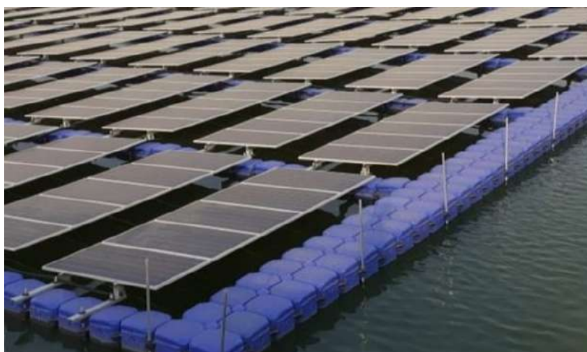
Figure 3- Showing floating Solar panels mounted fully in plastic
