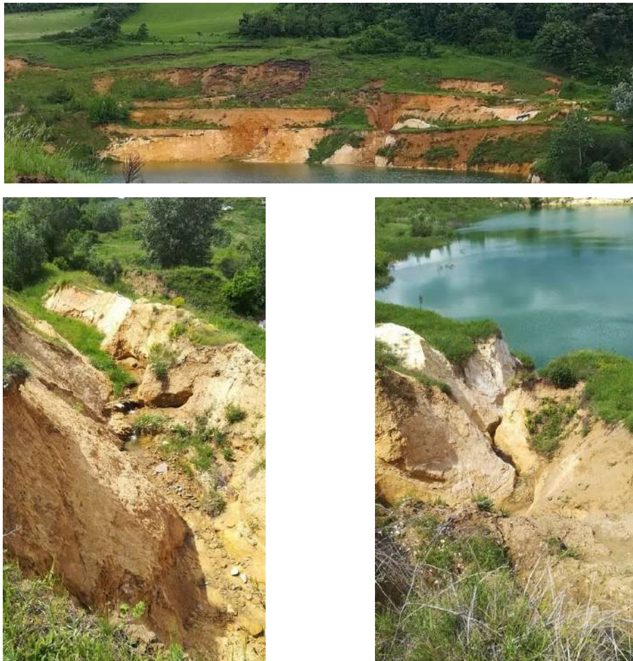
Figure 3 – Landslide in the south slope of VP2 and gully curved by Dulan stream
