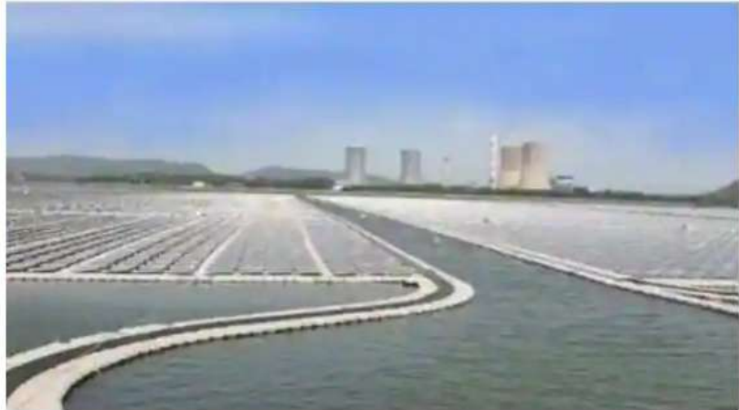
Figure 4- Showing Laying of floating Solar panels at NTPC Simhadri
