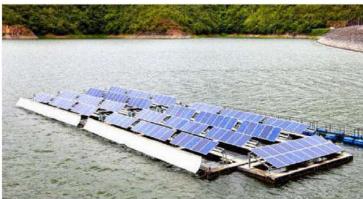
Figure 1- Showing Laying of floating Solar panels
